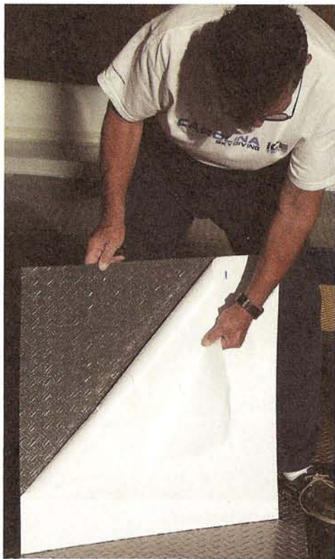
The peel-and-stick aspect of these tiles cuts down on the mess and clean-up factors of the project.
