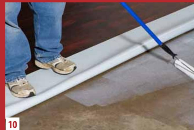
**10** Fold back the middle of the sheets to expose the unglued section of concrete. Apply adhesive, allow it to flash, and replace the flooring so that the edges meet. Smooth the floor with the heavy roller.
