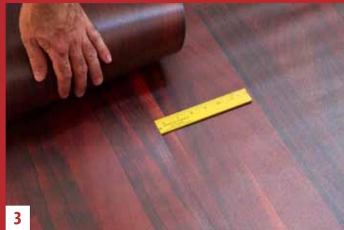
**3** Where you'll seam the flooring, roll out a second sheet overlapping the first by about 2 inches so you can cut them both later for a precise fit. Measure carefully to ensure the sheets run parallel to each other. Place heavy weights, such as a 5-gallon bucket half full of sand or water, on the flooring so that it will not shift.
