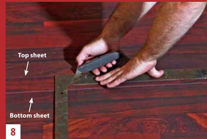
**8** Snap a chalk line down the center of the two sheets where they overlap. Cut through the overlapping sheets simultaneously, using a utility knife, and a straightedge such as a framing square.
