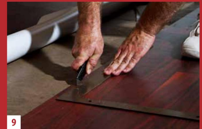
**9** If the utility knife cannot cut all the way through both sheets, fold the top sheet back and finish the cut on the bottom sheet. Take care to cut along the score line so that the seam between the two sheets meets precisely without gaps.
