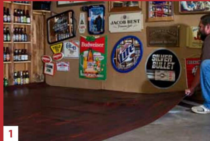
**1** After thoroughly sweeping the floor and vacuuming all dust and debris, dry-fit the floor along a side wall of the garage with the sheet rolled out from front to back. Allow the ripples of the flooring to "relax" and flatten for a few hours. Position the flooring so that it overlaps the wall by about an inch.
