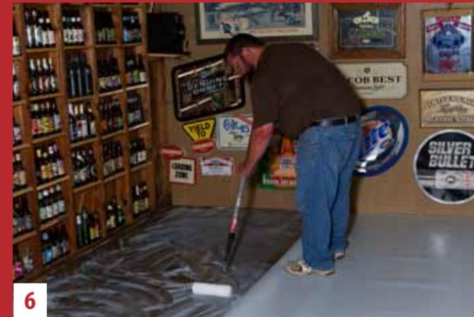
**6** Spread the adhesive with a paint roller that has been pre-loaded with extra adhesive. This ensures the roller does not take up adhesive but smooths out what has been applied with the trowel. Allow the adhesive to "flash" or dry according to the manufacturer's instructions before folding the flooring back into place.
