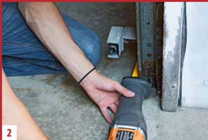
**2** Roll the flooring away from any obstructions that cannot be removed (such as garage-door tracks) and undercut them slightly higher than the thickness of the flooring. Remove any baseboards with care and reinstall them later.
