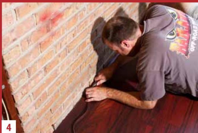
**4** After ensuring the floor has flattened and no folds or wrinkles appear in it, trim the floor around the walls with a utility knife. Change blades often to keep a clean cutline.
