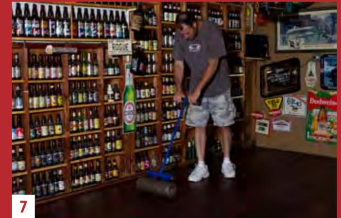
**7** Using a weighted roller, smooth from the center of the floor to the edges to force out any bubbles. Repeat Steps 5 and 6 for the second sheet. Then, follow the same procedure for the center halves of both sheets, applying adhesive to all but a 2'-wide section where the sheets overlap.
