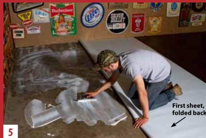
**5** Fold back half of the first sheet and apply adhesive, using a square-notched trowel recommended by the manufacturer.
