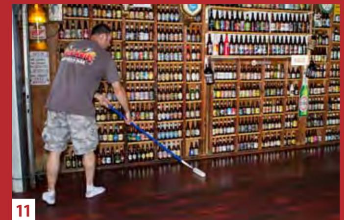
**11** Apply the finish recommended by the manufacturer according to its instructions to protect the floor and give it a gleaming finish.
